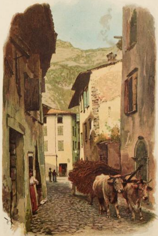
Straße in Vago.
